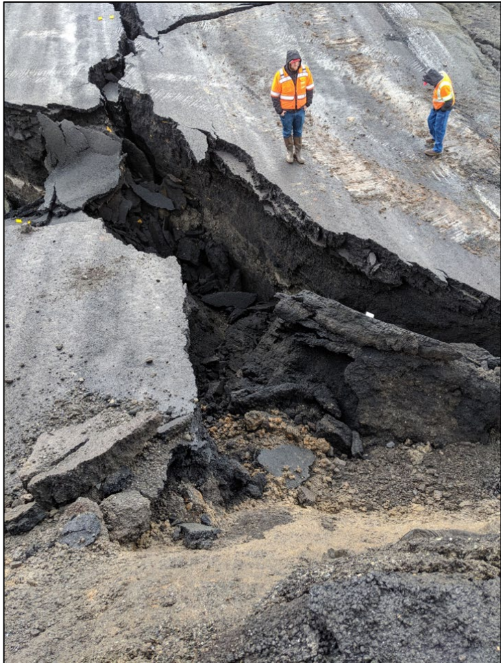
The February 2019 Hooskanaden Landslide closed U.S. 101 between Brookings and Gold Beach for two weeks. Rock from the proposed Colebrook Quarry could be used to help with future emergency landslide repairs.
